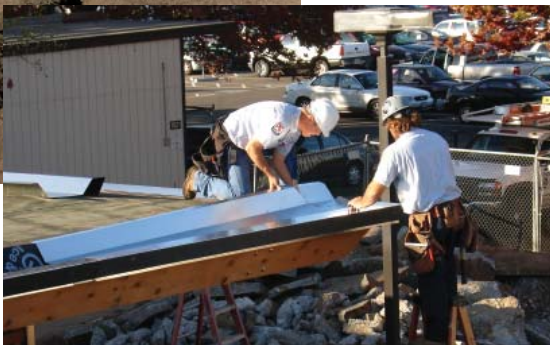
Below: Yuba College Building 1000 Roofing Installation
