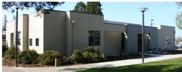
Below: DSPS Building at Yuba College
