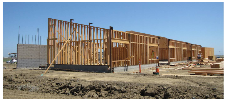
Above: Colusa County Outreach Facility
