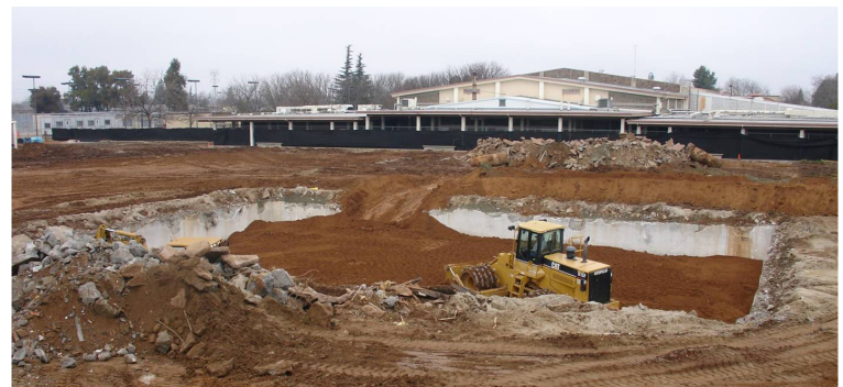
Below: Filling of the pool for the new athletic fields at Yuba College
