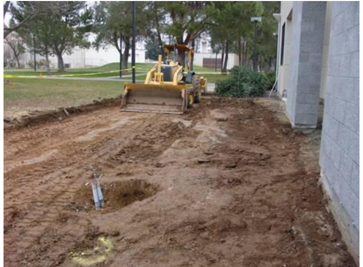
J-21 - Building 1800 ADA Renovations
