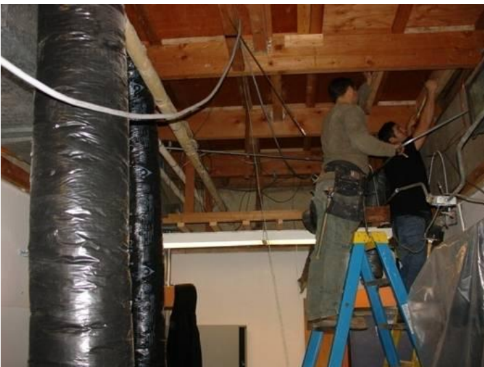
J-30 - IT Server Room HVAC Upgrades
