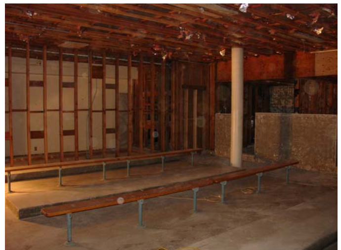
Hazardous Materials Abatement Complete PE Complex, Volume II, Yuba College
