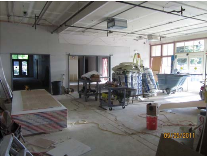
Building 100 Renovation in Progress Woodland Community College
