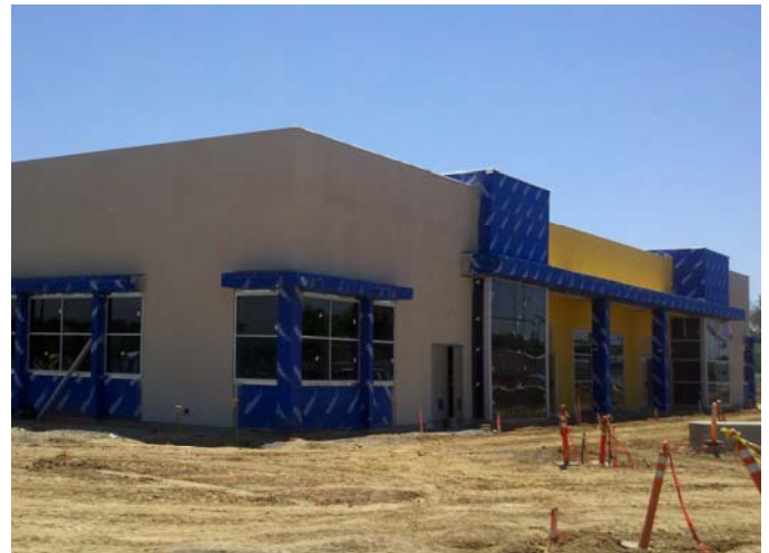
Construction Progressing Health & Public Safety Building, Yuba College
