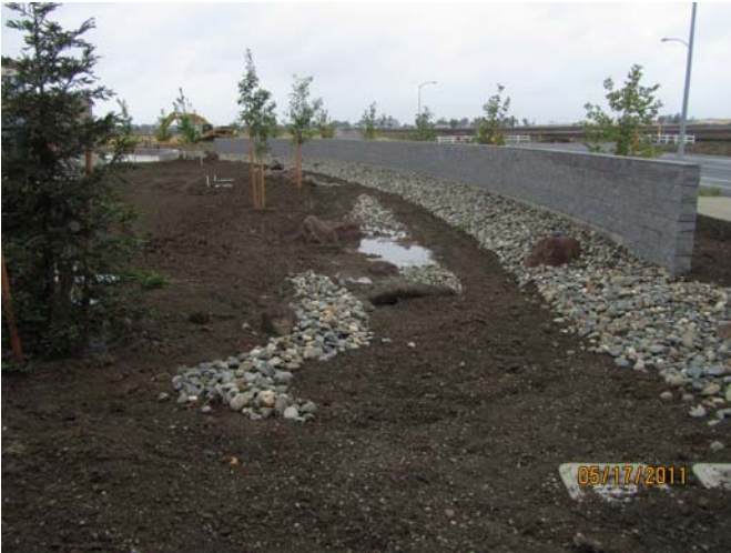
Landscaping Progressing, Woodland CC Colusa County Outreach Facility
