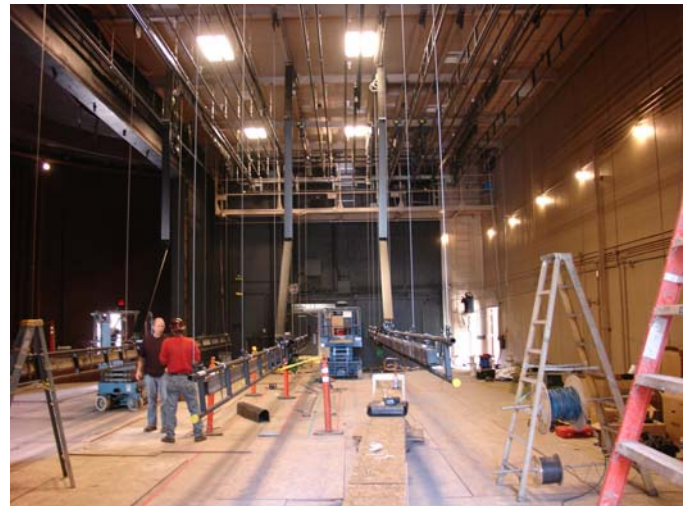
Stage Rigging Installation Building 400 Theatre, Yuba College
