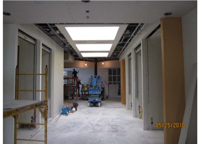
Interior Renovation Progresses Building 700, Woodland Community College
