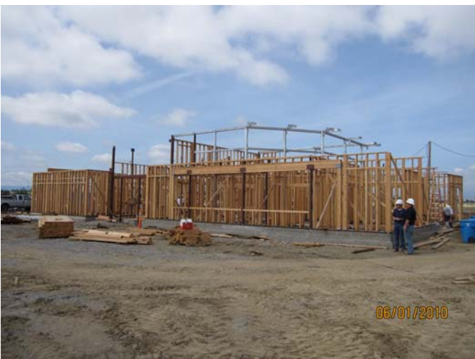
Foundation Work, Woodland Community College Colusa County Educational Outreach Facility
