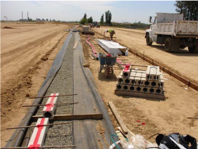
Field Perimeter Drainage Installation Athletic Fields, Yuba College
