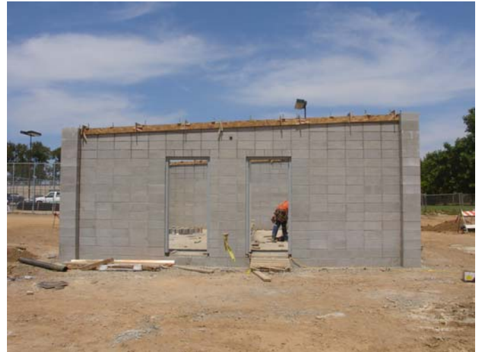
Building C Construction Continues Athletic Fields, Yuba College
