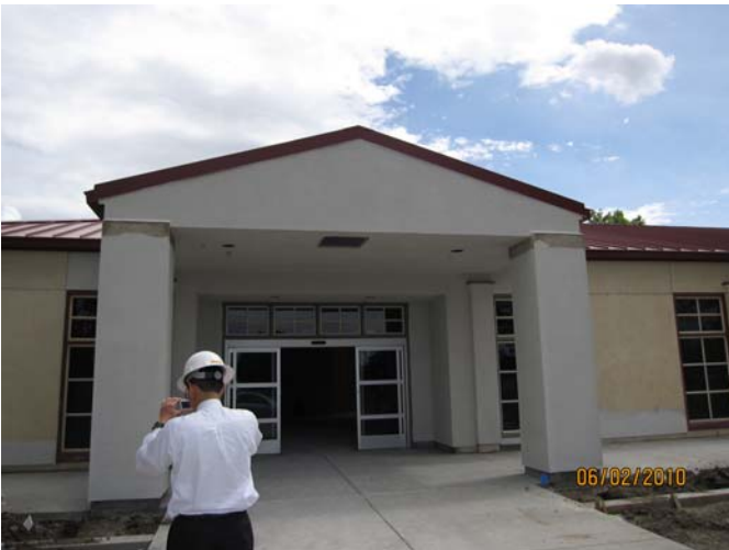
Exterior Renovation Nearly Complete Building 700, Woodland Community College
