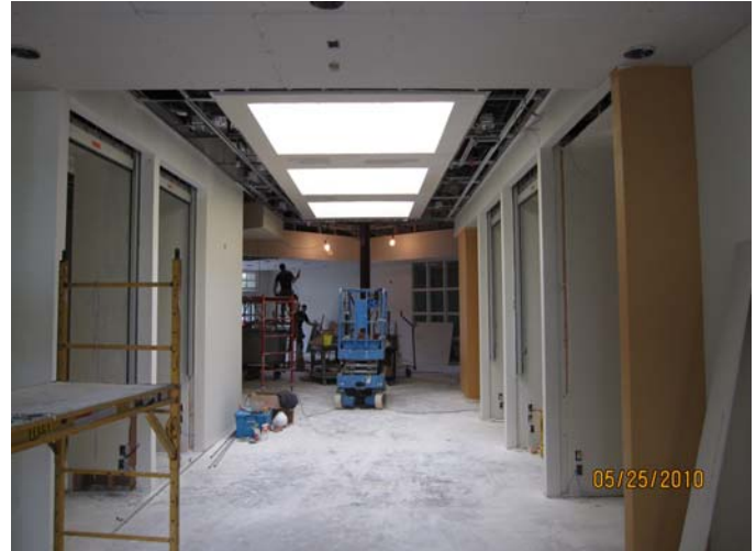
Interior Renovation Progresses Building 700, Woodland Community College
