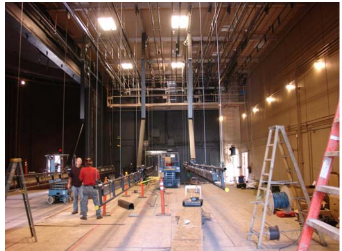
Stage Rigging Installation Building 400 Theatre, Yuba College
