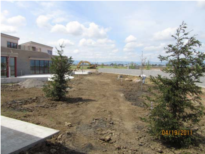
Landscaping work started, Woodland CC Colusa County Outreach Facility
