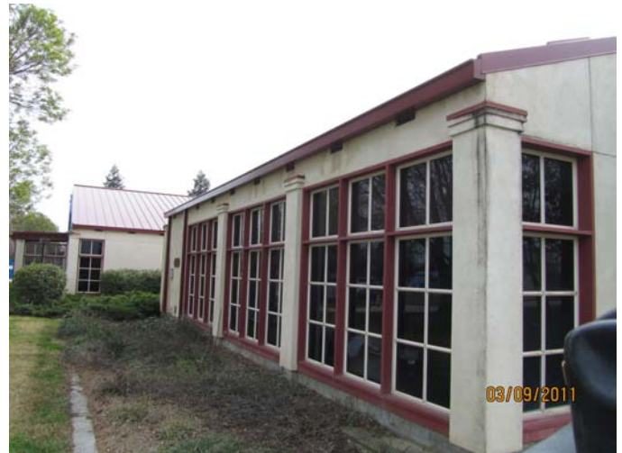
Building 100 Re-Roof Complete Woodland Community College
