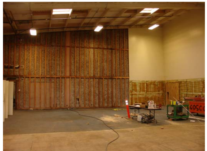
Building 1200 Renovation—New Matt Room PE Complex, Volume II, Yuba College
