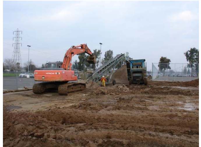
Construction Demolition Continues Athletic Fields, Yuba College
