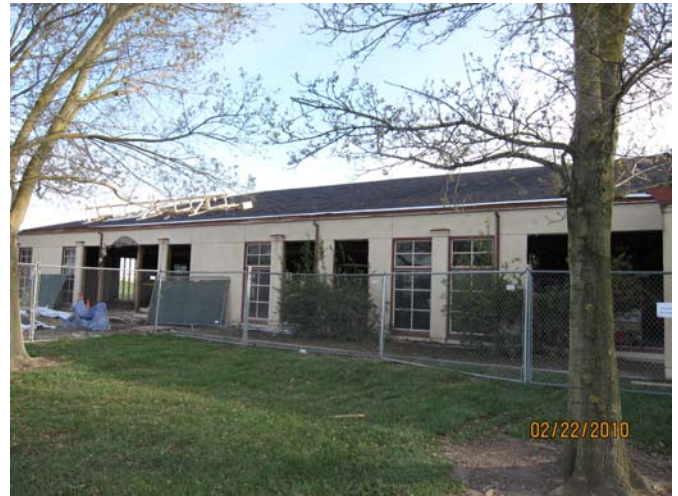
Exterior Renovation in Progress Building 700, Woodland Community College
