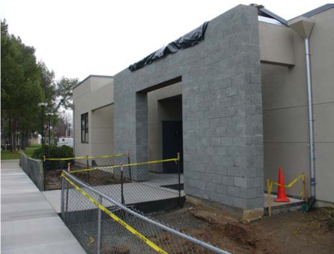
Exterior Renovations Building 1800 DSPS, Yuba College
