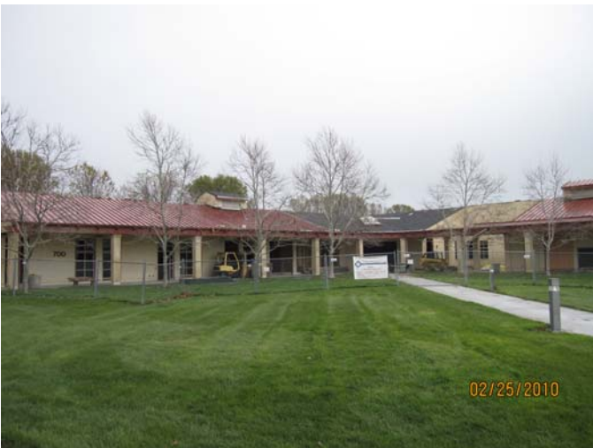
Exterior Renovation Begins Building 700, Woodland Community College
