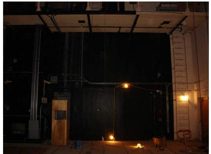
Interior Renovations Building 400 Theatre, Yuba College
