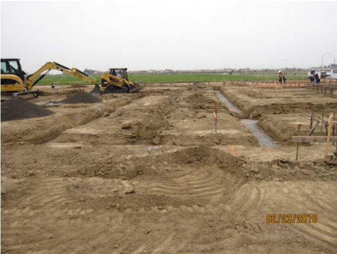
Site Work, Woodland Community College Colusa County Educational Outreach Facility
