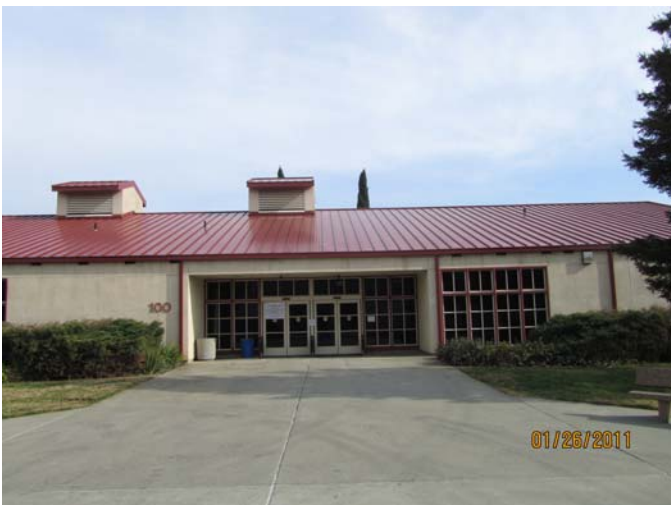
Building 100 Re-Roof Complete Woodland Community College
