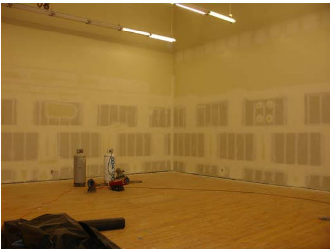
Building 1200 Renovation—Weight Room PE Complex, Volume II, Yuba College
