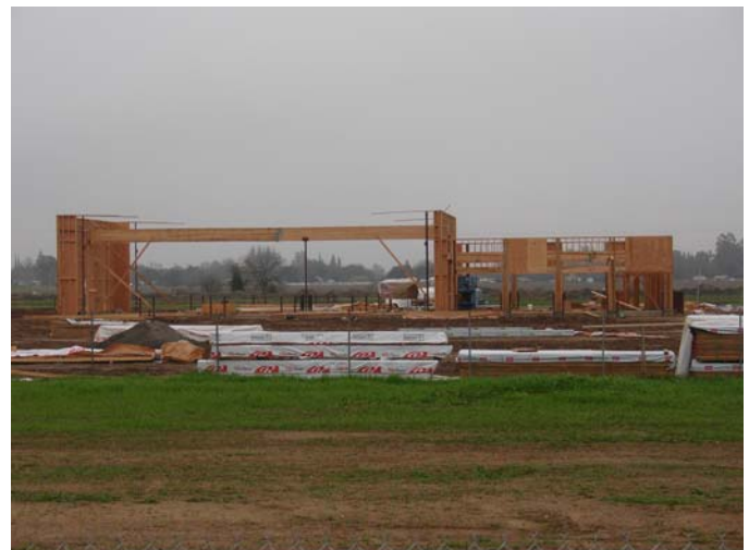
Vehicle Service Building, Yuba College Health & Public Safety Building
