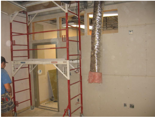
Campus Police Relocation, Construction in Progress Woodland Community College
