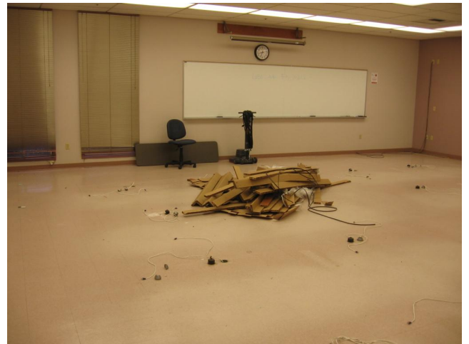
Geology Lab Renovation, Start of Demolition Woodland Community College
